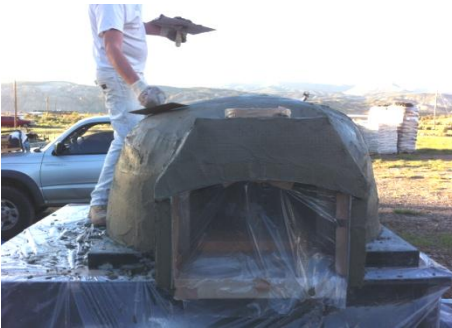
Putting on the stucco
